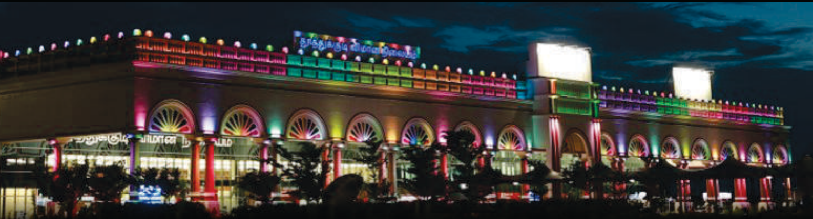
Fig. 1 — The Passenger Terminal Building's colonnaded façade under a multi-hue dynamic lighting scene. Individually addressable RGB fixtures wash each fan-lit arch in a different hue, while a continuous parapet cove line traces the building's full elevation.
