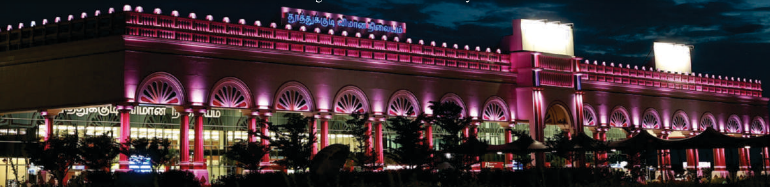
Fig. 2 — The same elevation reprogrammed to a monochromatic magenta scene. Demonstrating the system's full-spectrum colour-changing range, this scene shows how a single hue can unify the cove line, arch washes and column lighting into one cohesive, saturated composition — useful for festival, brand or occasion-based lighting scenes.
